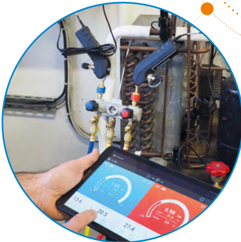
PERFORM CHECKS WITH THE SI-RM13 COMBINED MANIFOLD
