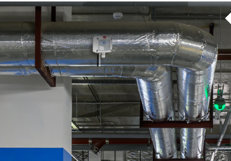
The CP 112 connected to a Debimo device mounted in a ventilation duct. Our Debimo accessories for air flow measurement on page 17.
